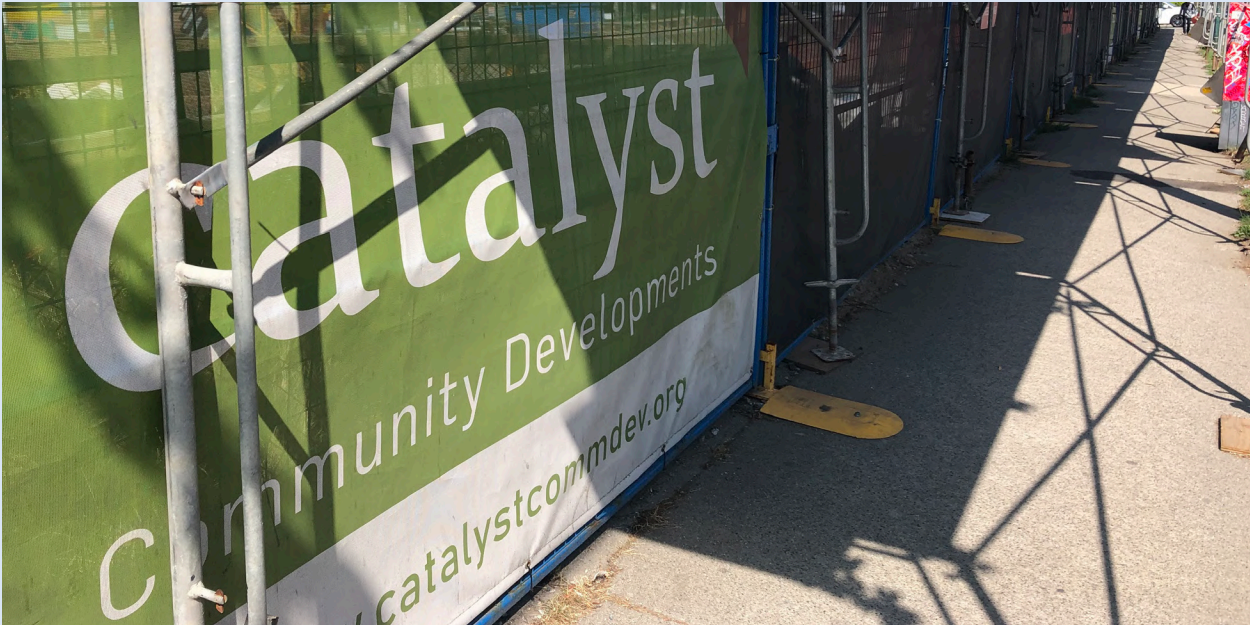
Construction site of 2221 Main St redevelopment project. Photo Credit: Jean Roe
